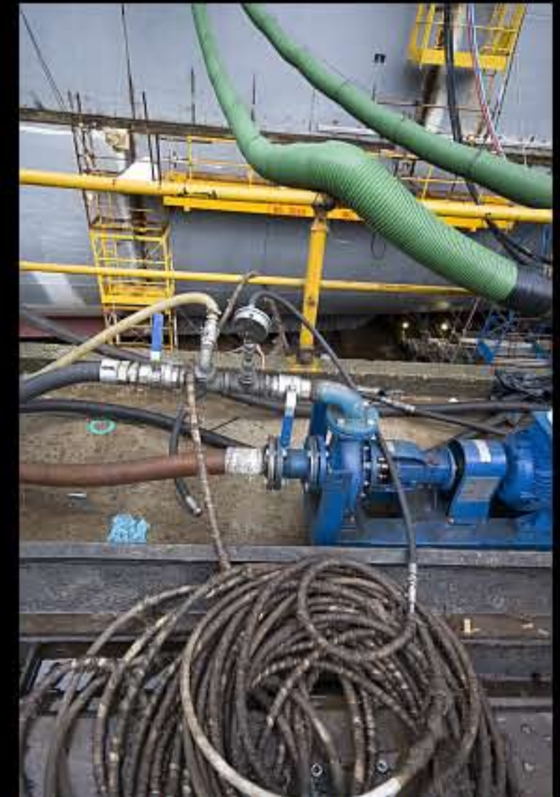
Italy, Venice, Marghera industrial district, Fincantieri Marghera-535
