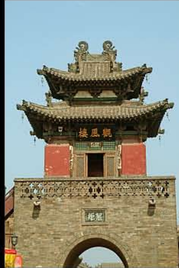
Pingyao, Tingyu Building
